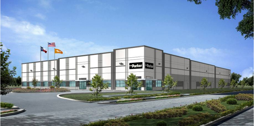
Photo Cutline: Parker Corporation Energy Products Division Headquarters
